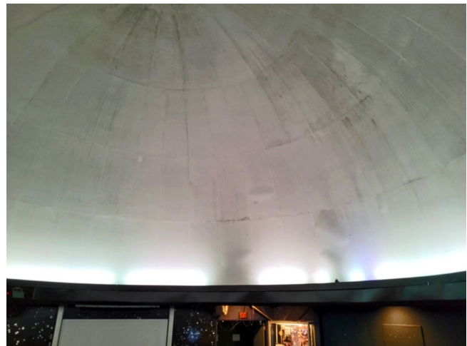
The recent fire at the Ward Beecher Planetarium seriously damaged its dome, speakers, cove lights, and interior. Photographs submitted by Curt Spivey.
