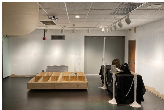
Walls being prepared for a vinyl wrap and the insert wall being prepared to be installed within the double-door opening.
